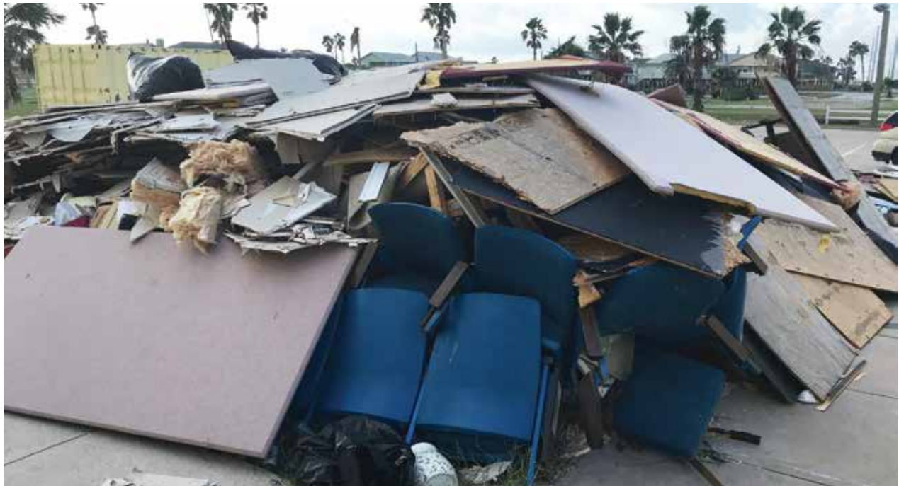
After more than a decade of hosting theatre patrons, PACT's flood-damaged auditorium seats had to be removed and discarded along with interior walls, subflooring, and carpeting
